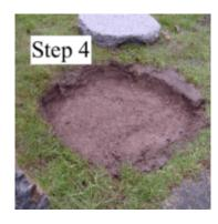
4. Dig out some soil to create a pocket for the bed of mortar. The top of the stepping stone should finish below the level of the lawn when completed.
