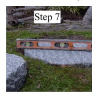
7. Use a spirit level to ensure that the stepping stone is at the correct height and that it is laying level. Allow the bed of mortar to cure for one or two days before using the path.
