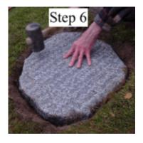
6. Lay the stepping stone on to the mortar and hammer down with a rubber mallet.
