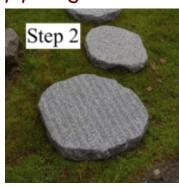
2. Lay the stepping stones out to ensure that they are in the correct position. The stepping stones should be set with their centres around 55cm apart.
