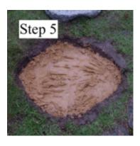
5. Prepare a mix of four parts 'soft sand' and one part cement with some water. The bed of mortar should be around 5cm thick to ensure a solid base.
