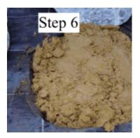
6. Prepare a mix of four parts 'soft sand' and one part cement with some water.The bed of mortar should be around 5cm thick to ensure a solid base. Lay the stepping stone on to the mortar and hammer down with a rubber mallet.
