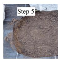
5. Mark around the stepping stone and cut out the weed membrane. Dig out some soil to create a pocket for the bed of mortar, allowing sufficient space around to move the stone if required.
