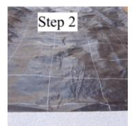
2. Lay weed membrane over the area. Fold the edges under, and pin it down.
