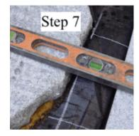
7. Use a spirit level to ensure that the stepping stone is at the correct height and that it is laying level. Allow the bed of mortar to cure for one or two days before using the path.
