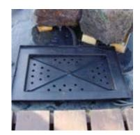
7. Place the tank lid/mesh over the opening and cover the liner with water worn cobbles, slate, mulch or gravel.
