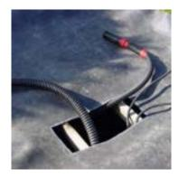
4. Put the pump into the tank, and connect the hose pipe. Take the electrical cables out of the tank for connection to the power supply.
