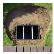
2. Dig a suitably sized hole for the water tank. Ensure that it is level. Profile the soil around the tank forming a shallow basin with the tank at the lowest point.
