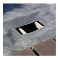
3. Lay the piece of liner over the tank leaving a 'skirt' all the way around. Cut a letter box slot in the liner directly over the center of the tank. Make it just big enough to get the pump through.
